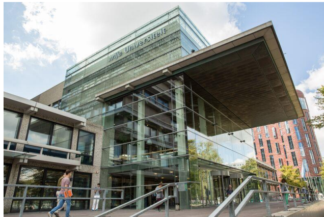
VU campus main building
